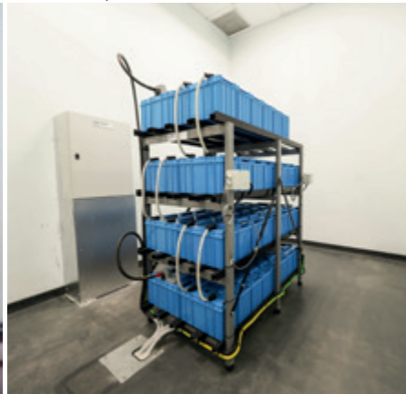
Example with 16 batt packs, Total output: 116kWh
