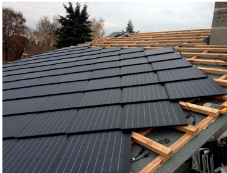
... the tiles are laid from the eaves to the ridge ...
