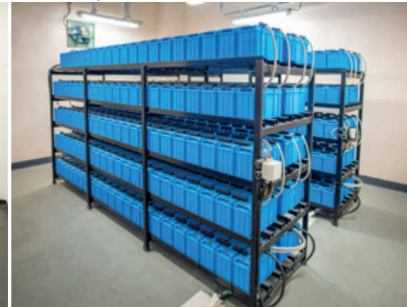
Example with 110 batt packs, Total output: 792kWh
