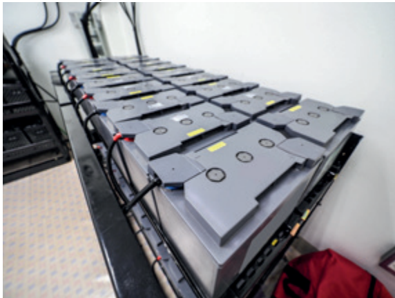
Example with 4 batt-packs, Total output: 28.8kWh
